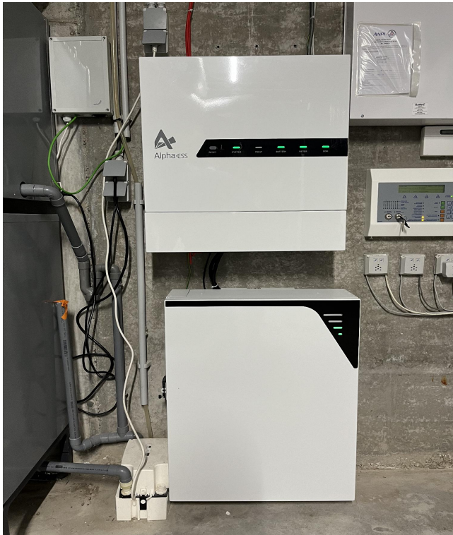
Figure 6: HomeLab battery used for testing the proposed control framework in real world
